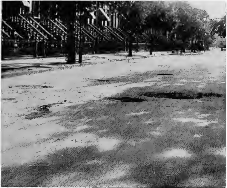
JEFFERSON AVENUE, BROOKLYN, 1900. Destructive effects of gas leaks on sheet-asphalt pavement.
